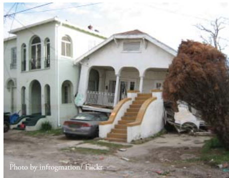
The result of a soft story collapse.
